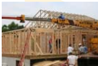
Roof trusses being put into place on the Perry home.
